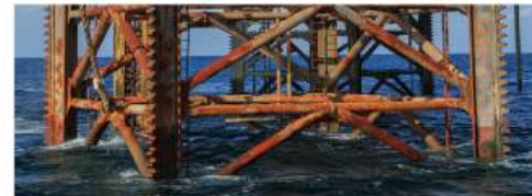
ABS Group, Jack-Up Drilling Rig, 2025
